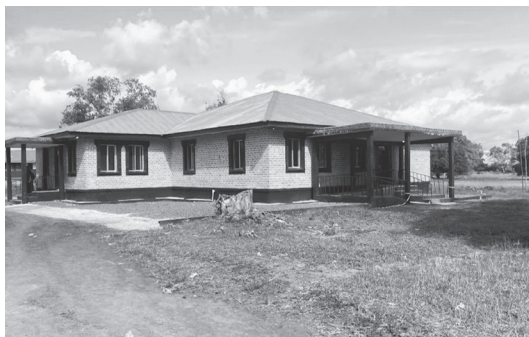
This newly renovated health clinic at Ricks Institute in Liberia will serve the students and the surrounding community.
